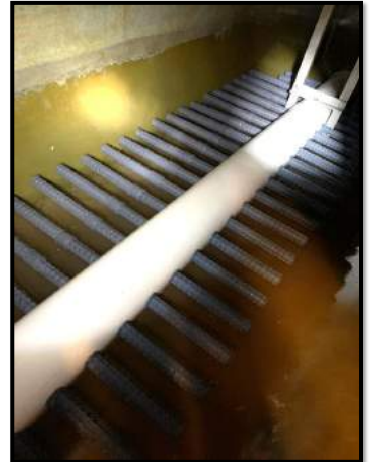
New Lateral in sand filter
