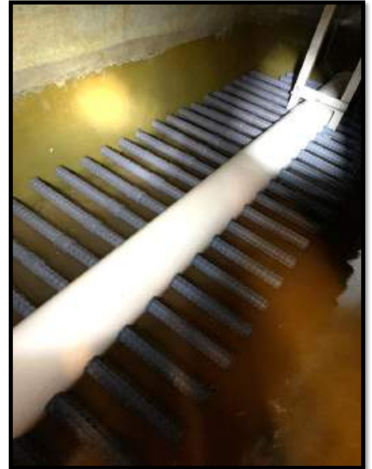
New Lateral in sand filter
